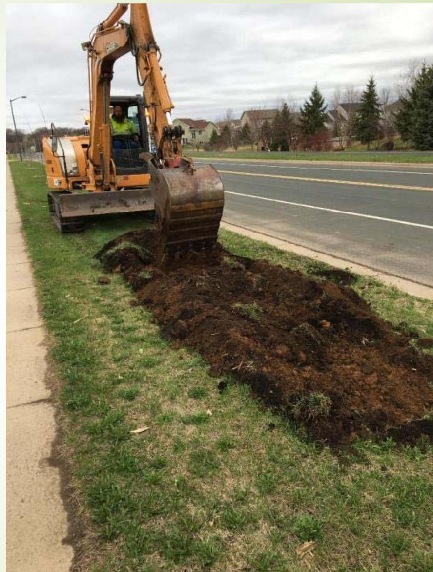
This is an example of the “scoop and dump” method of preparing soil, and incorporating some compost into the soil in the process. Large bed plantings like this are best done with a backhoe.
